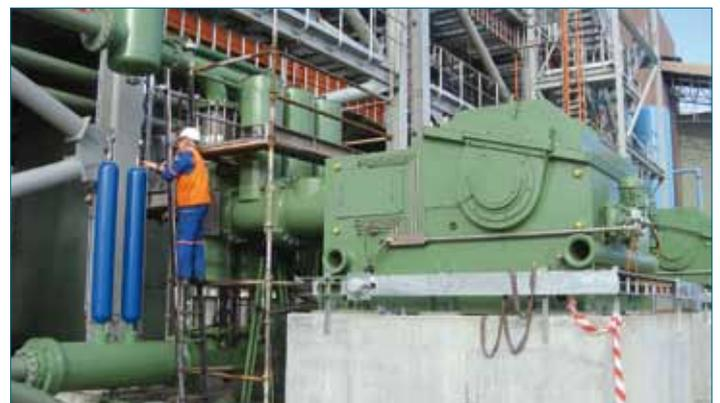
Fig. 8: Double hose-diaphragm pumps in triplex design
